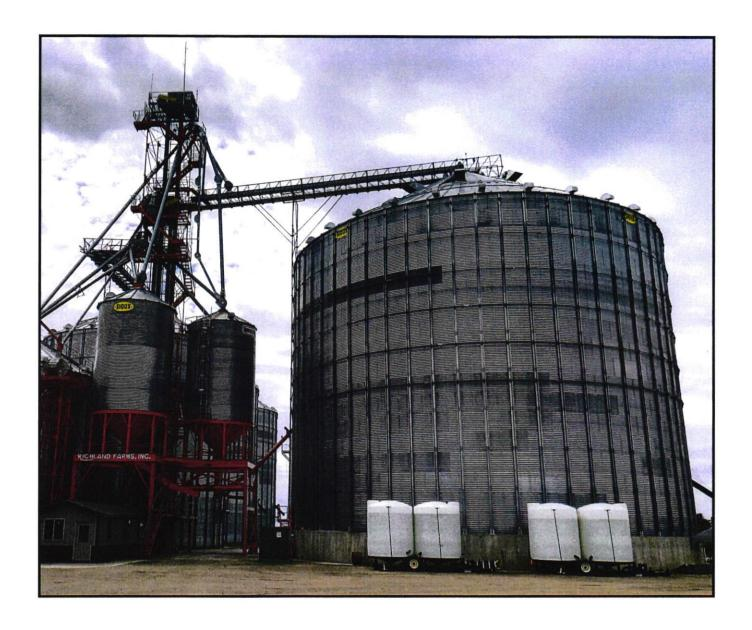
Grain storage setup includes three 60x62 feet and one 96x66 feet. Each has metal sides, rod and concrete foundation. The larger bin tunnel with unloading drag underneath. The smaller bins have individual unloading augers will require utilization of a portable auger for unloading. The capacity of the subject bins at 56 pound test weight level full is approximately 900,000 bushel.
