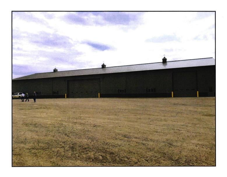
Machine shed is  $72 \times 208 \times 18$  feet. This is a pole metal morton building constructed 2011/2012. There is 20 foot concrete apron on the east side.
